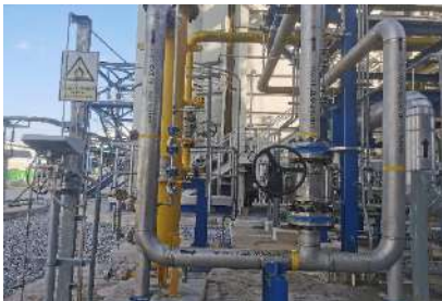
FG filter Block valve (isolate point2)
