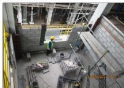
Block wall and lintel-stud work of BRH room
