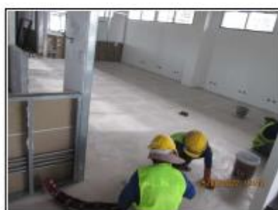
Cement grouting the granito floor tile at 4th fl.
