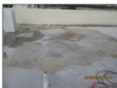
Self leveling of roof slab.
