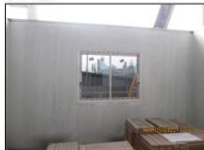
Install the aluminum-glass window at operator room level +7.50.
