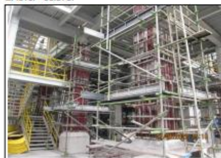
Installation the column formworks at ground fl.
