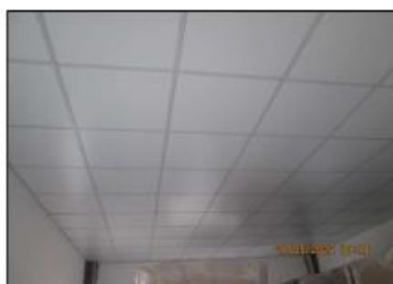
Installation the t bar gypsum ceiling of DCS room +13.50.
