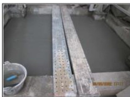
Pouring the slab concrete at lift pit.
