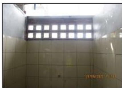
Ventilation block wall work at toilet +13.50.
