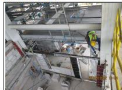
Block wall and lintel-stud work of BRH room
