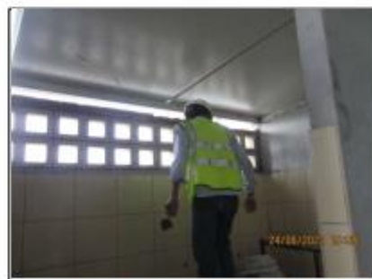
Ventilation block wall work at toilet +13.50.
