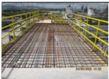
Installation the wiremesh and block out slab at level +38.375.
