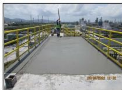
Pouring the concrete slab at level +38.375. grid line C-D/1'-1
