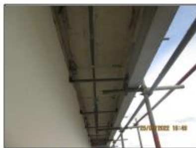
External aluminum ceiling frame at staircase roof slab.
