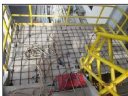
Installation the landing wiremesh at stair ST-2.
