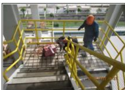
Installation the landing wiremesh at stair ST-2.
