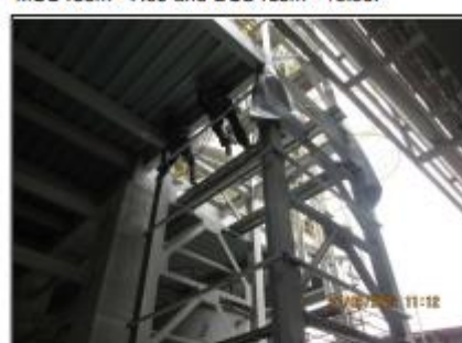
Installation the siding metal sheet frame of elevator steel structure.
