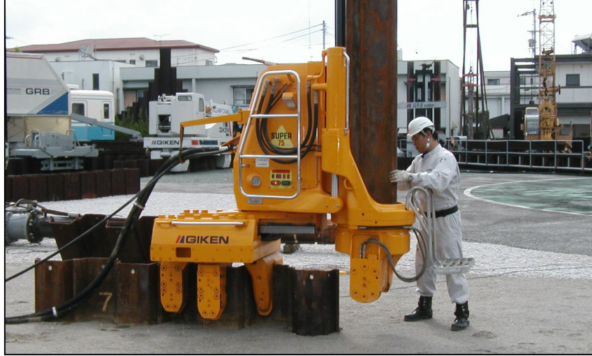
Figure 1 Installation of sheet piles using the press-in method
