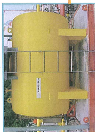
2114 D-004 HIGH EXPANSION FOAM CAPACITY 2.5 M3 LEVEL 50- 85 %
