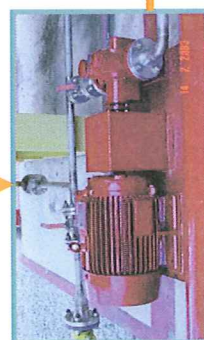
2114-P-005 HIGH EXPANSION FOAM PUMP DISCHARGE PRESSURE 18.5 BARG
