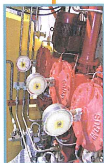
2114 Y-004.5.6 CONCENTRATE CONTROLLER HIGH EXPANSION FOAM 3 % MIXING 3%
