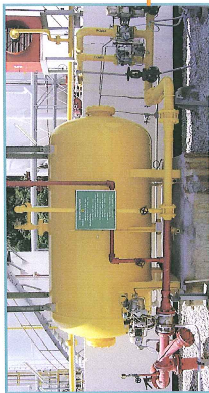
2114 D-002 LOW EXPANSION FOAM CAPACITY 3.7 M3 LEVEL 50- 85 % AFFF 3%
