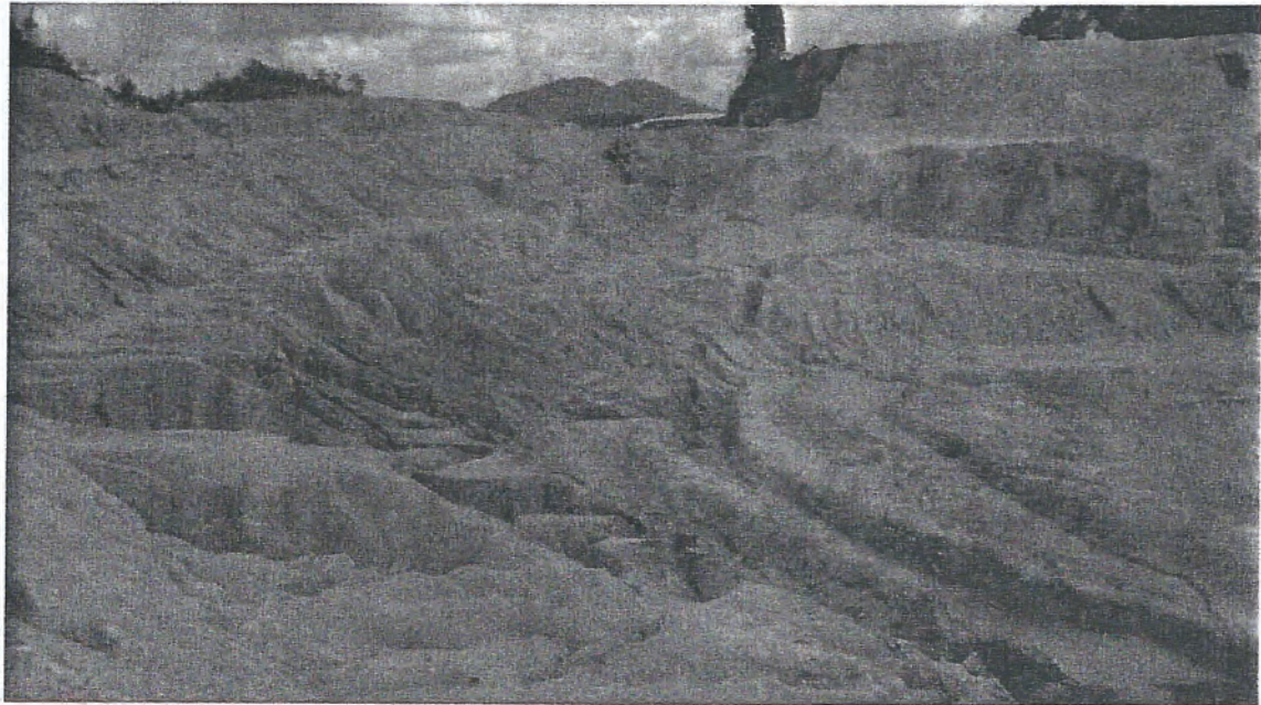
Figure 10 Slope failures due to erosional process at MRD mine.
