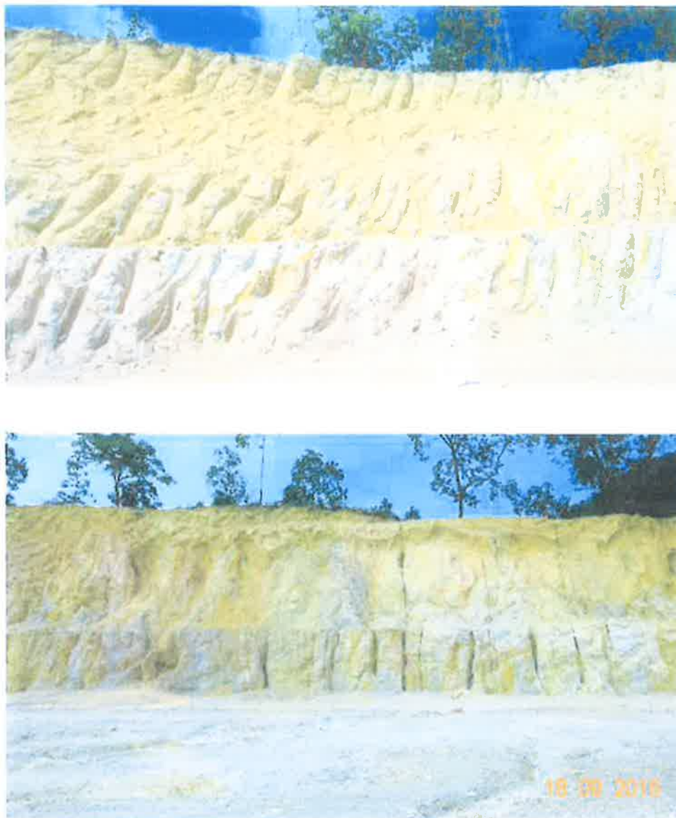
Figure 3 Pit slope before and after several small to big rainfalls.
