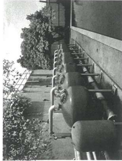
Automatic Sand Filter Capacity: 400 m 3 /hr
