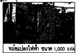
TRANSFORMER 1,000 KVA 33KV/400-230V. 3P, 50Hz
